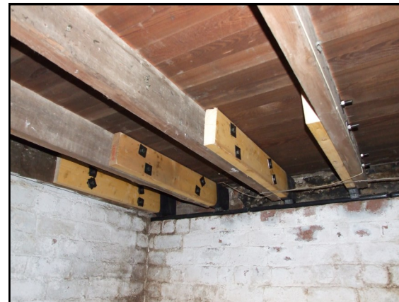
Main floor beam repairs in basement
